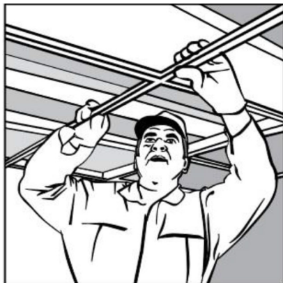
3. Installing the suspended grid
